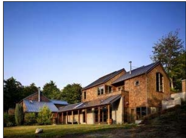
BENJAMIN BENSCHNEIDER / THE SEATTLE TIMES The newly remodeled and more-than-doubled-in-size house is pushed back into the hillside, roofed in metal and finished in shingles to blend into the island landscape.
